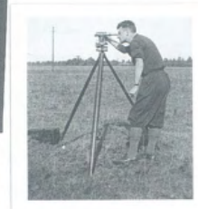
Survey work on Defford Common
